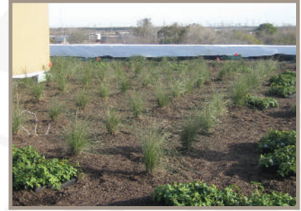
Green roofs provide many benefits — one being a recreation area for occupants.
